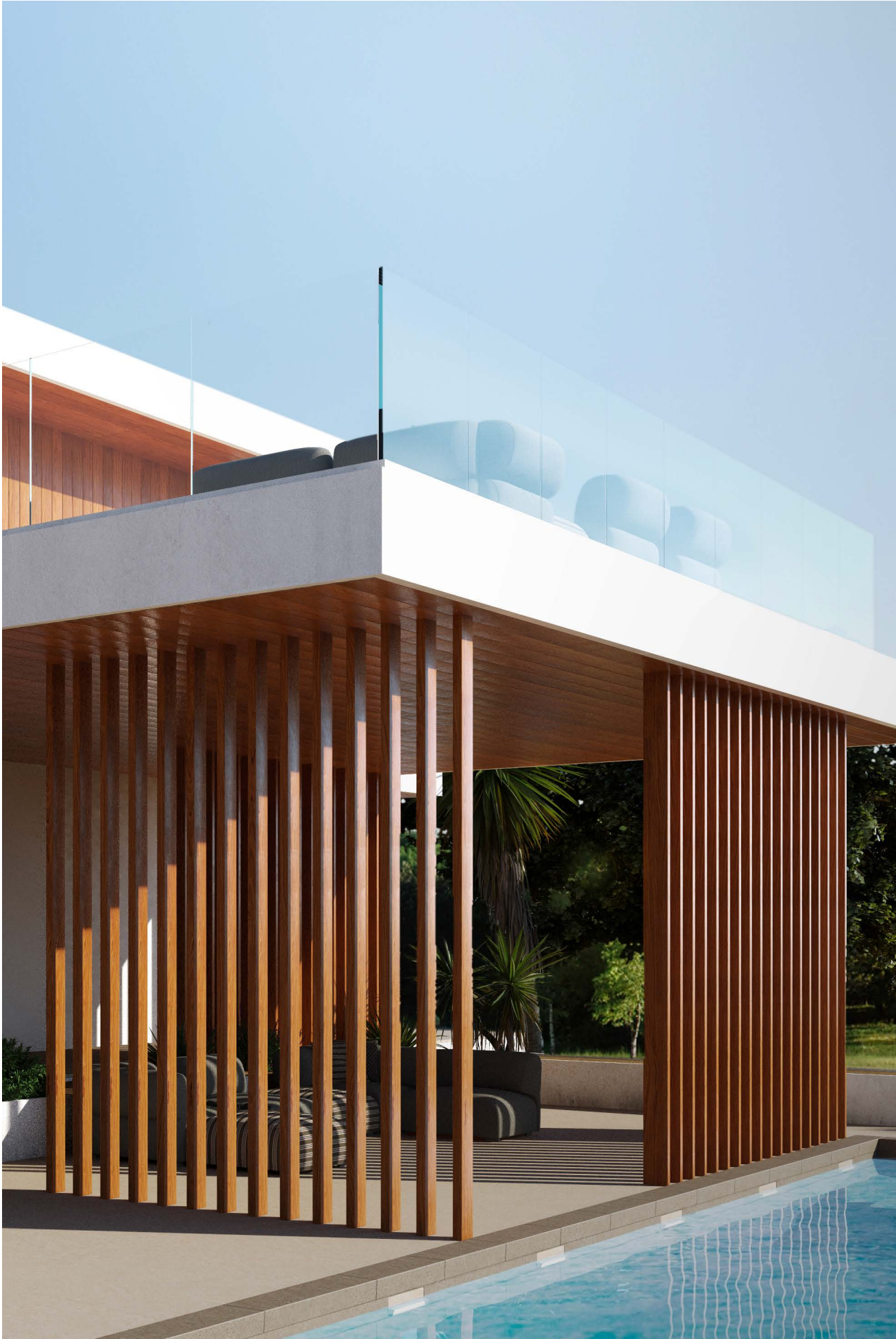
PRIVACY SCREEN EXTERIOR
